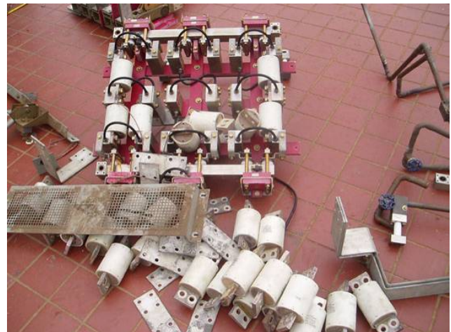
Figure 8. Old disconnect switch and fuses removed
