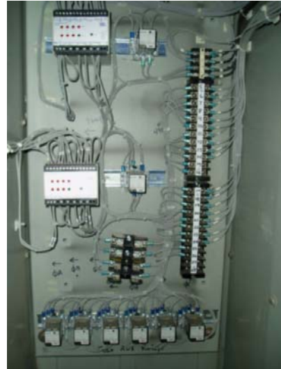
Figure 10. Temperature Relays and Remote Annunciation
